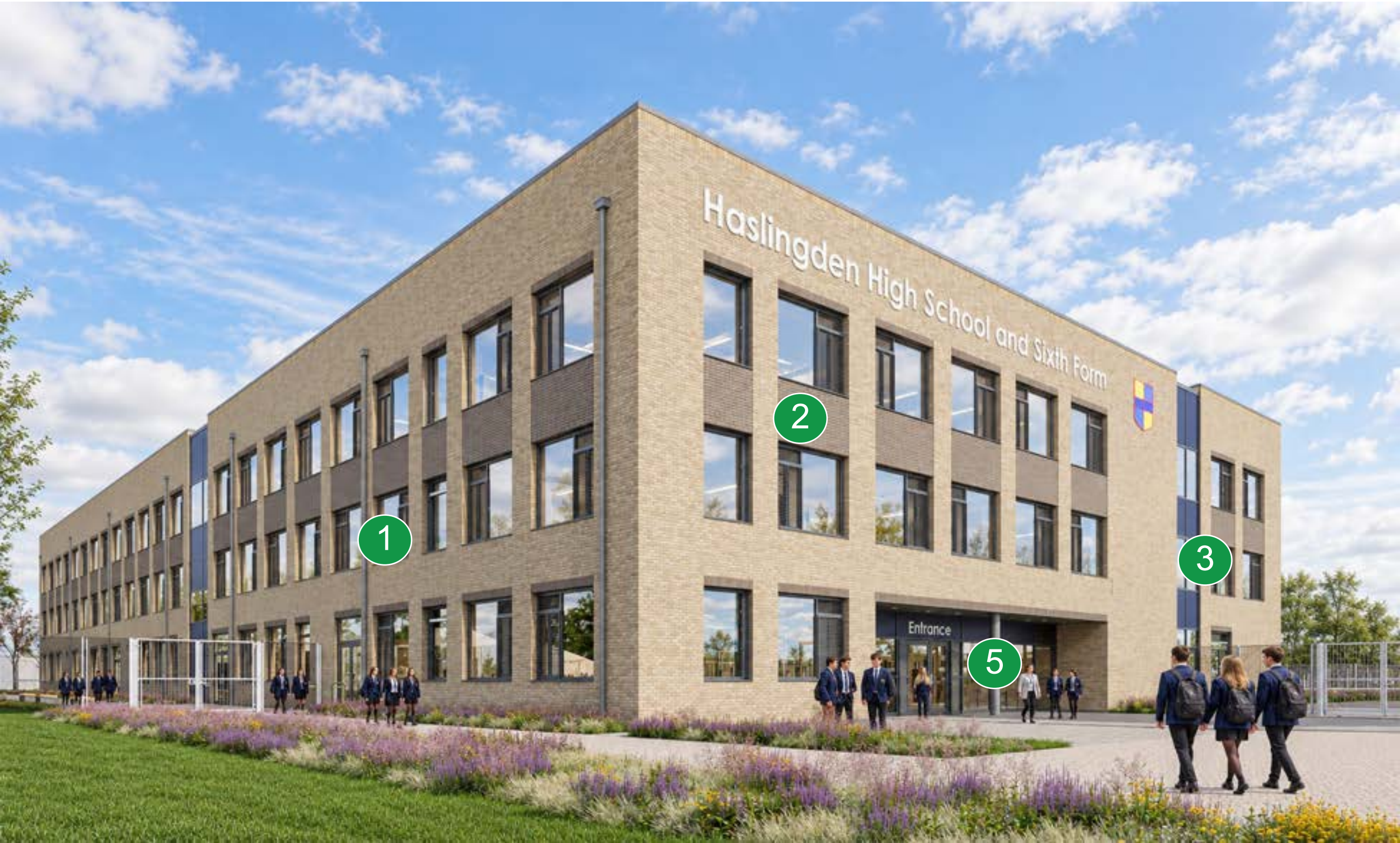
Main entrance (top left), sports-hall cladding detail (top right) and Broadway facade (lower right)
